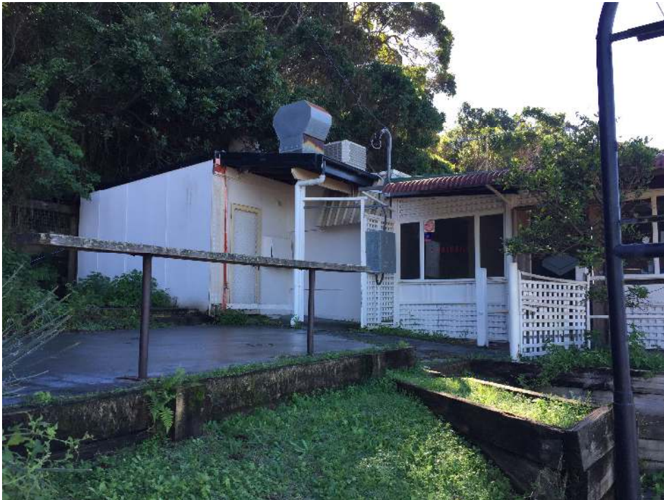
Image 2: A view from the south-western corner of the property towards entrance of the restaurant.
