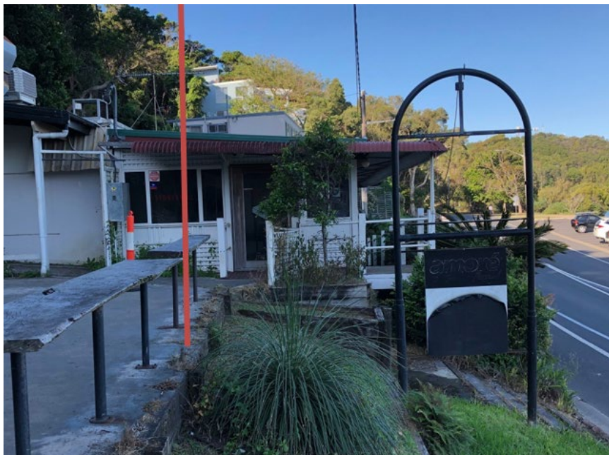
Photo 1 – View along western elevation of building on Lot 3 and footpath (red line indicates approximate location of front boundary).
