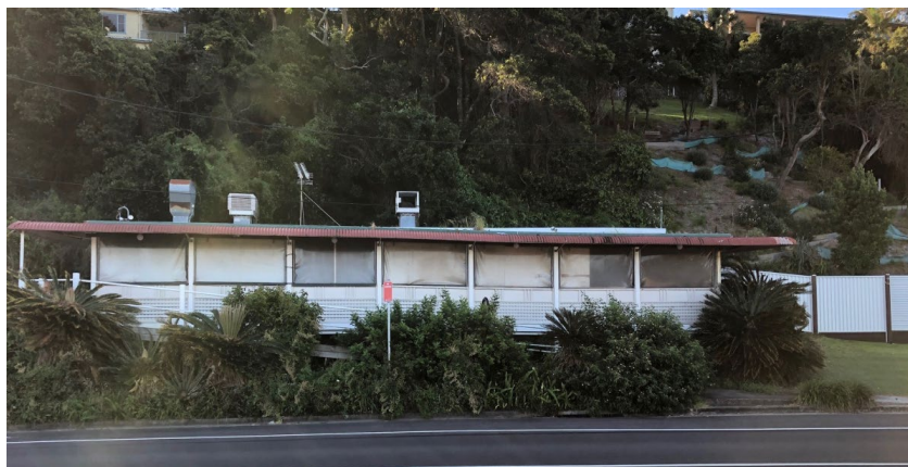
Photo 3 – northerly view from Compton Drive towards Lot 3
