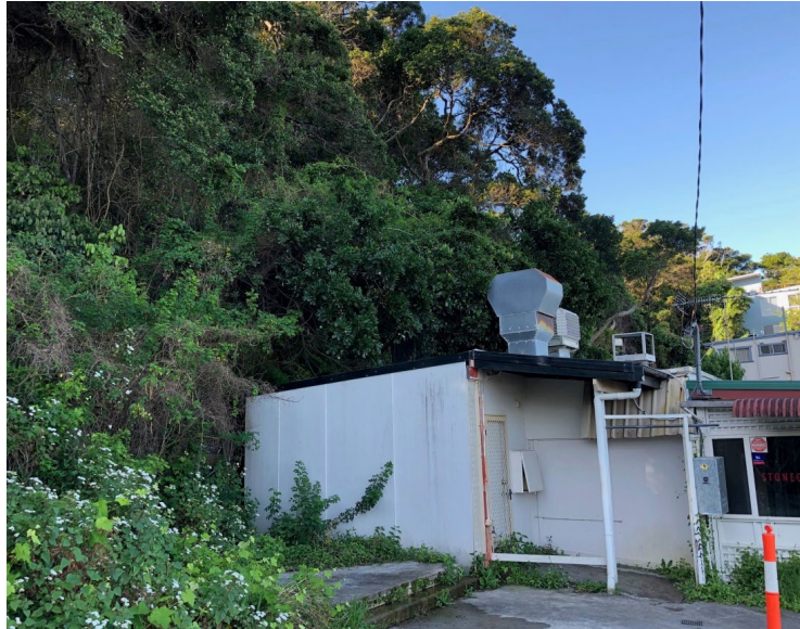
Photo 2 – view to the east from Lot 1 to Lot 3.
