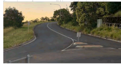
View looking up Ballina Heights Drive to the North.
