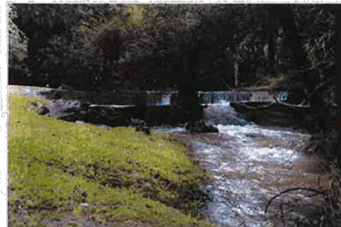
Bulwinkel Weir in flood, May 2015
