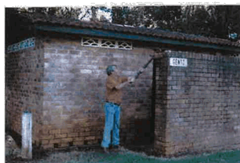
Lions Club doing maintenance on Toilet Block, 1990
