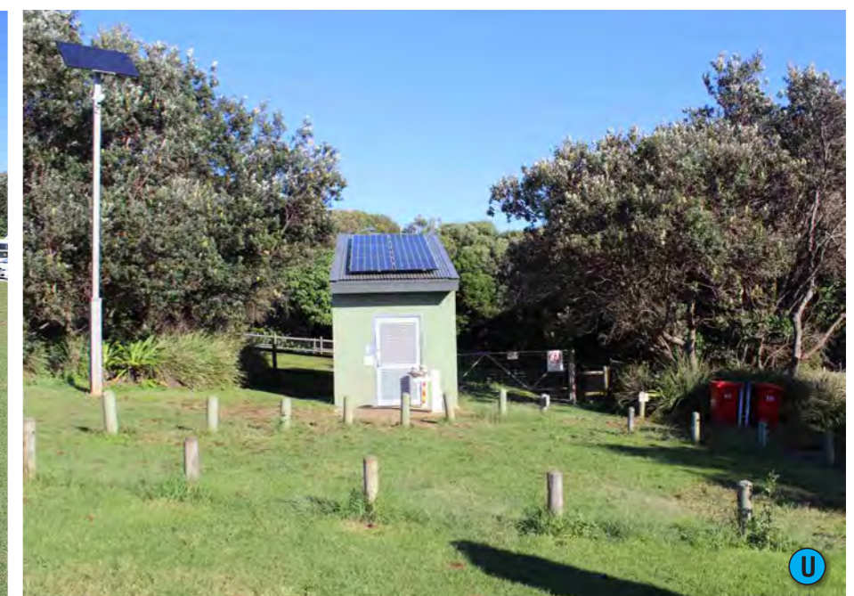
Above: The toilet building which is not legible as a public toilet. The effluent field is behind.
