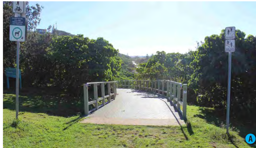
Above: Existing boardwalk component of the shared pathway that connects the Pat Morton Lookout Precinct to Lennox Head Village Centre.
