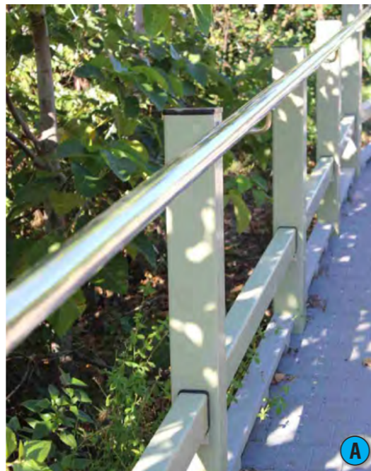
Above: Existing boardwalk construction
