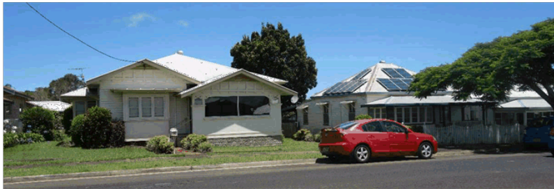
Views of the historical facades to residences at Nos. 10 to 16 The Avenue.
