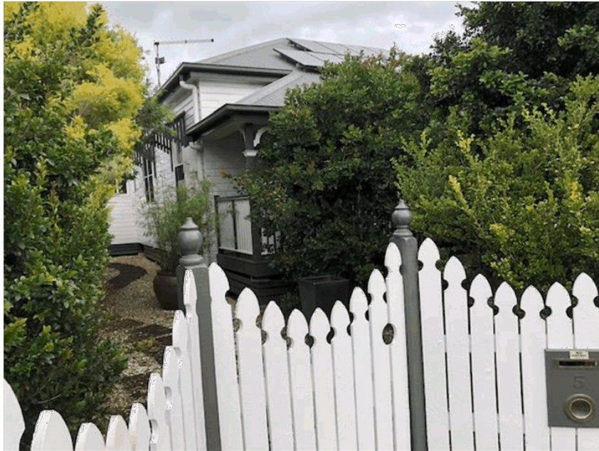
5 Daley Street single storey timber / iron roof dwelling
