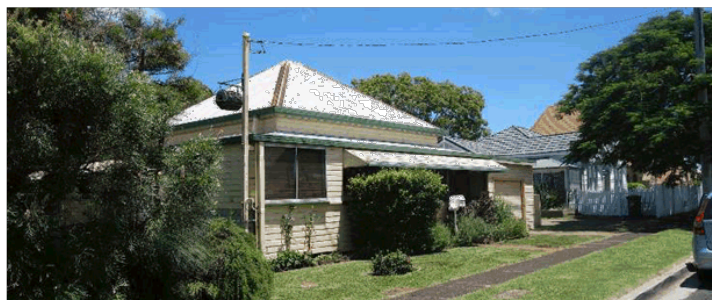
Although outside of the study area and with a commercial zoning, the above historical residences at 2 and 4 The Avenue should be considered for inclusion in the heritage conservation area.
