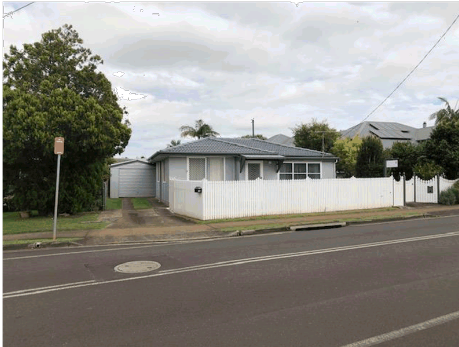
5A Daley Street single storey fibro and tile roof.
