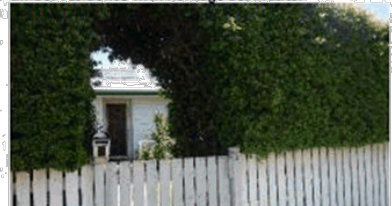
No. 3 Daley Street is hardly visible behind the picket fence and hedge.
