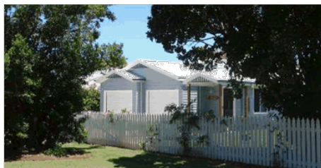
No. 1B 'Craven Cottage' is adjacent to No. 3 and while recent, has complementary façade elements and the white picket fence.
