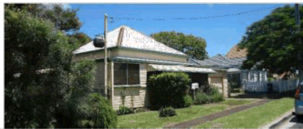
Although outside of the study area and with a commercial zoning, the above historical residences at 2 and 4 The Avenue should be considered for inclusion in the heritage conservation area.
