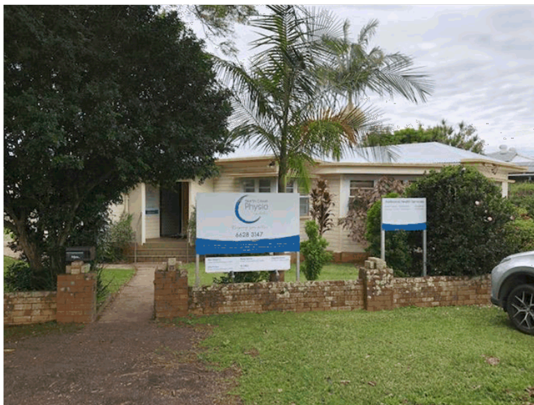
2 Daley Street within B2 zone
