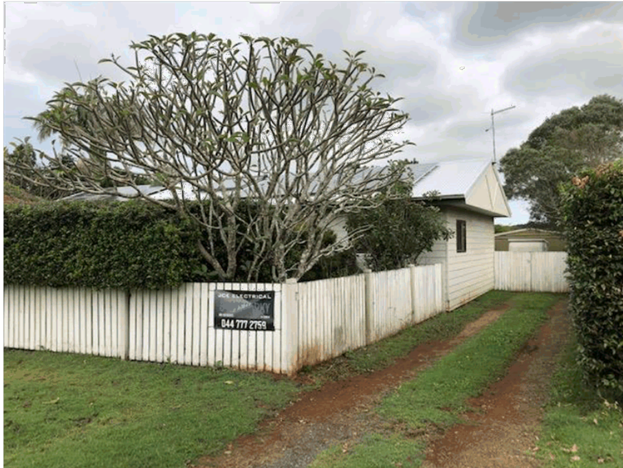
3 Daley Street – Picket fence approved in 2003. Compressed cement boards and gable end on building may indicate that this dwelling is not the original dwelling on this site.
