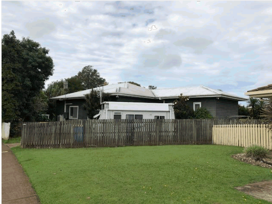
9 Daley Street crn Wardell Road single storey timber dwelling with iron roof.
