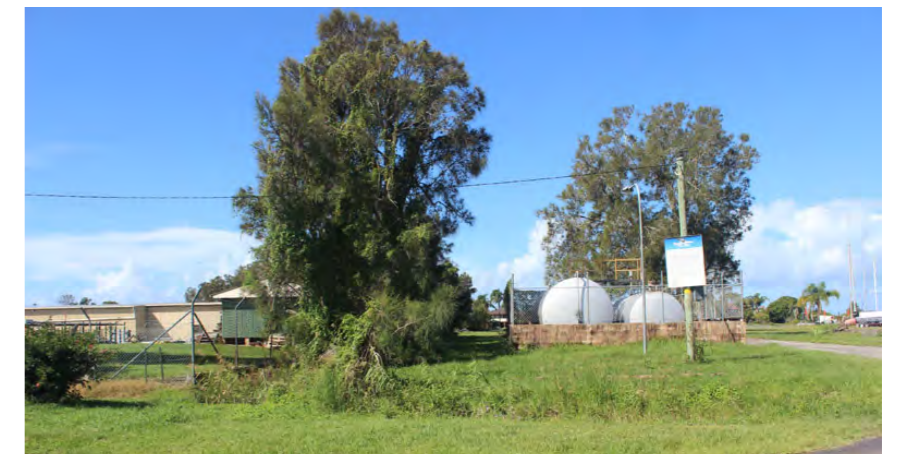
L existing fuel storage and southern extent of RMS depot
