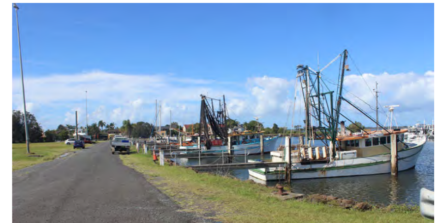
K vehicular access northern side of harbour
