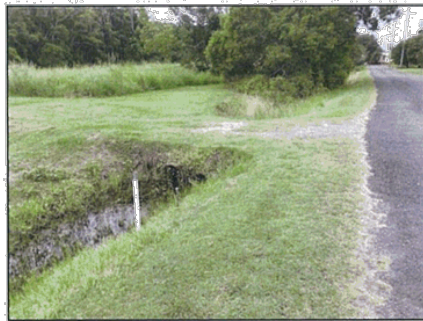
Photo 5 - Table drain within the road reserve.
