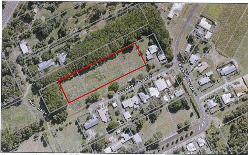
Figure 9—Existing access to Fitzroy Street
