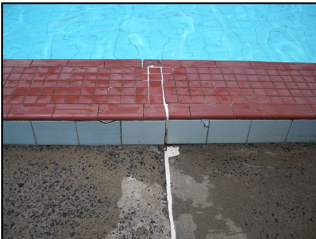
Pool Coping Tiling
