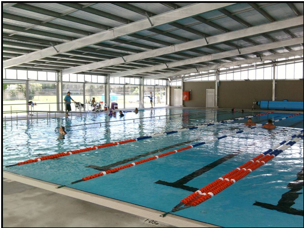
Coffs Harbour 25 metre Indoor Swimming Pool November 2010
