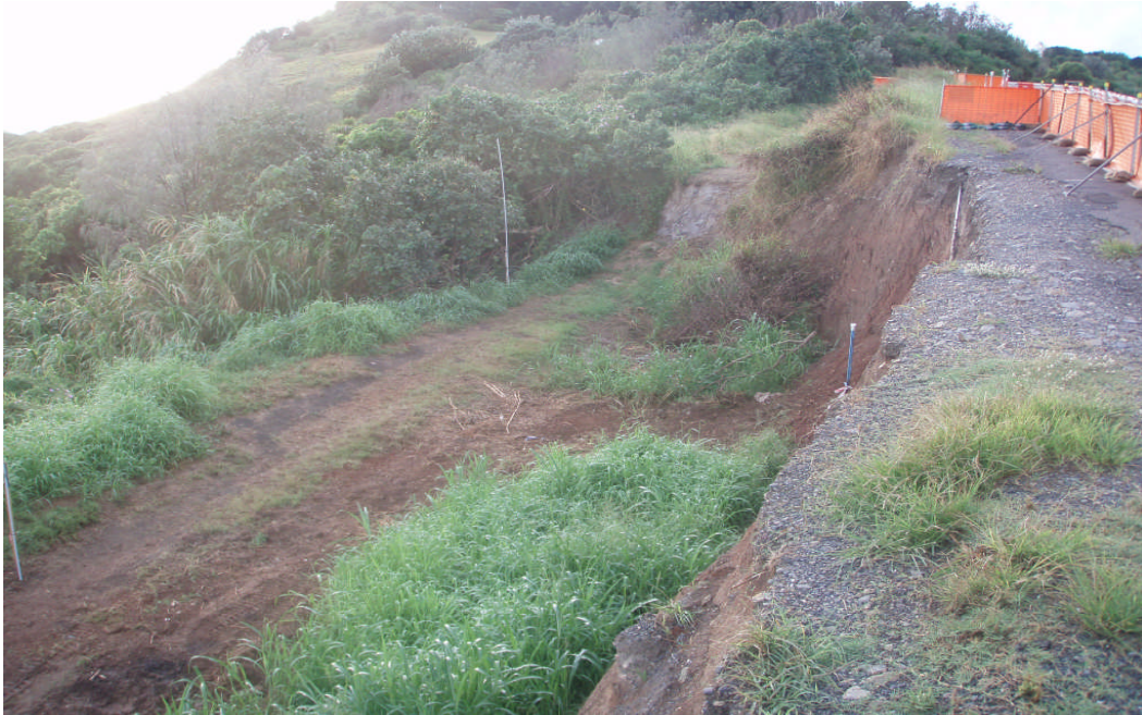
Photo 3: View of landslide head scarp and edge of road pavement, looking south east.
