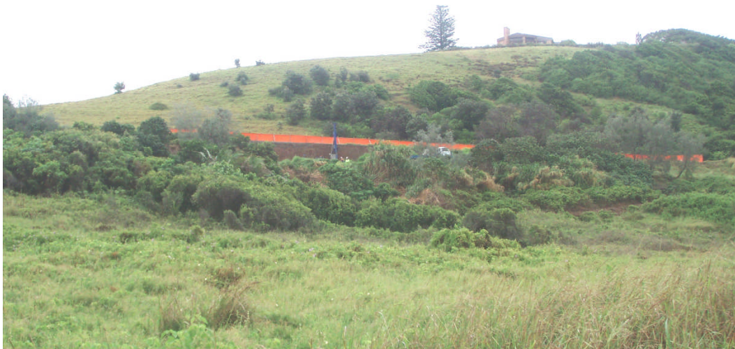
Photo 2: Regional view of Coast Road and the landslide area, looking west.
