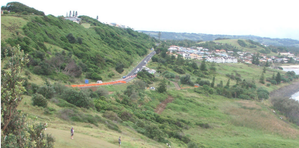
Photo 1: Regional view of Coast Road and the landslide area, looking north west.
