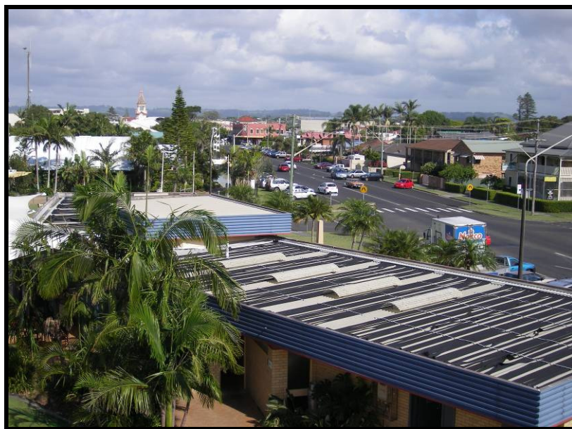
Pool Heating on Amenities Roofing
