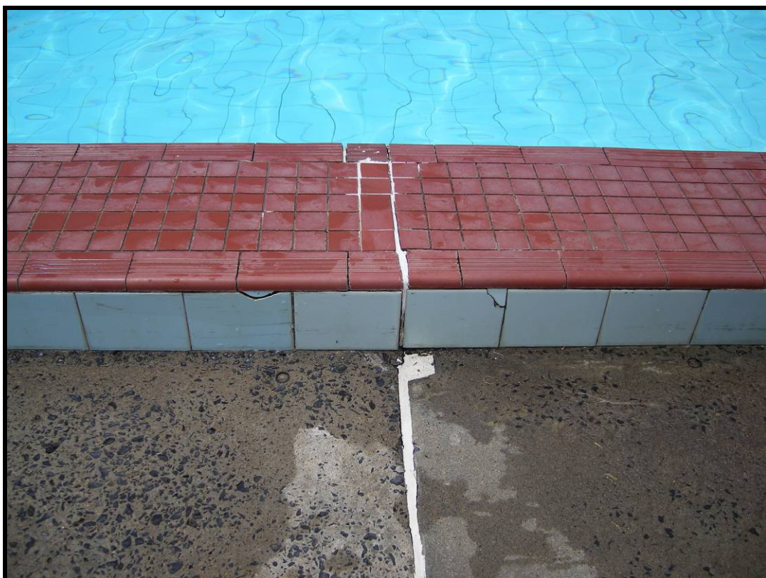
Pool Coping Tiling
