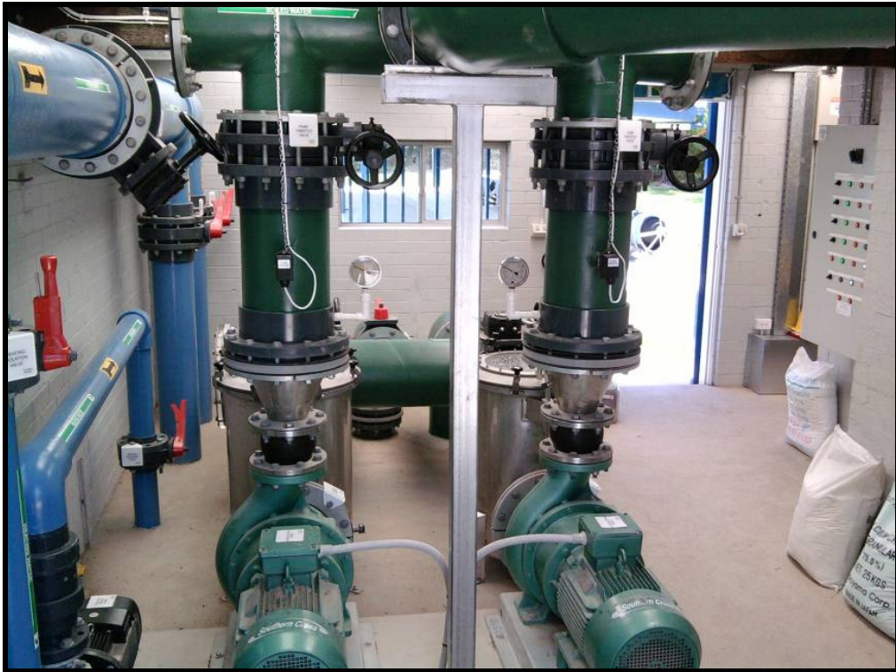
Coffs Harbour Pool Plant Room (November 2010)
