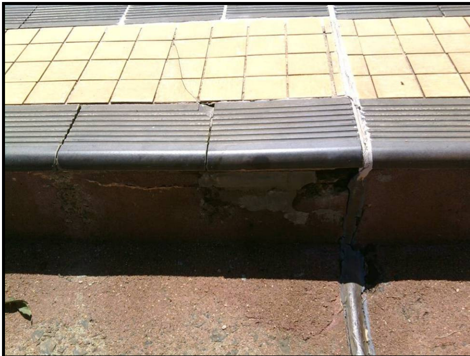
Sample of the Alstonville Pool Coping and Tiles
