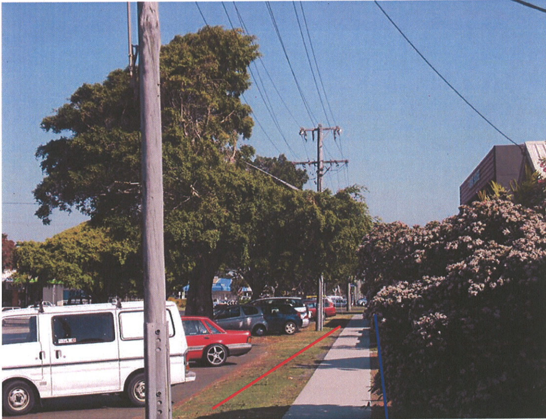
Photo 2: Red line indicates the only available position for a root barrier that does not interfere with services. Blue line indicates position that root barrier should be placed to ensure minimal impacts on trees.
