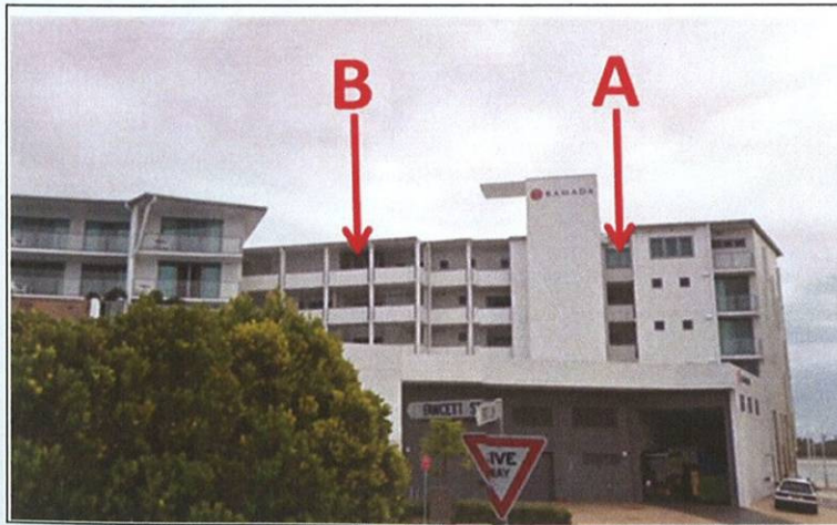
Figure 2: Photograph of north façade Showing glazing referred to in the text
