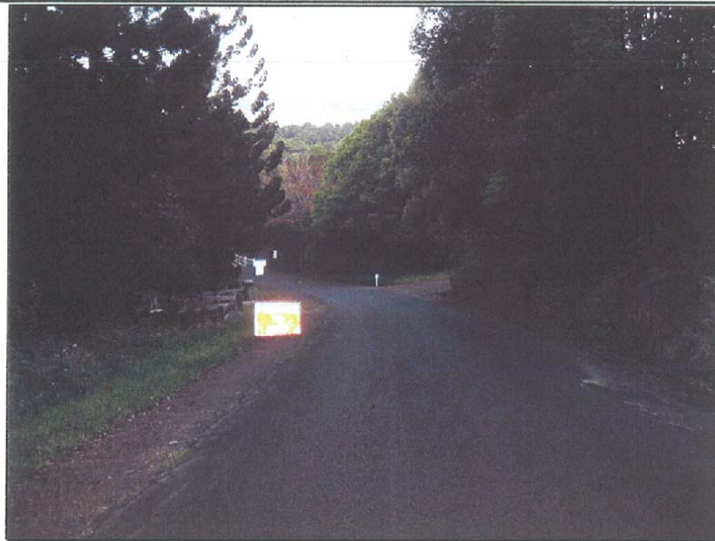
Figure 2 - Eltham Road north of Gibsons Creek
