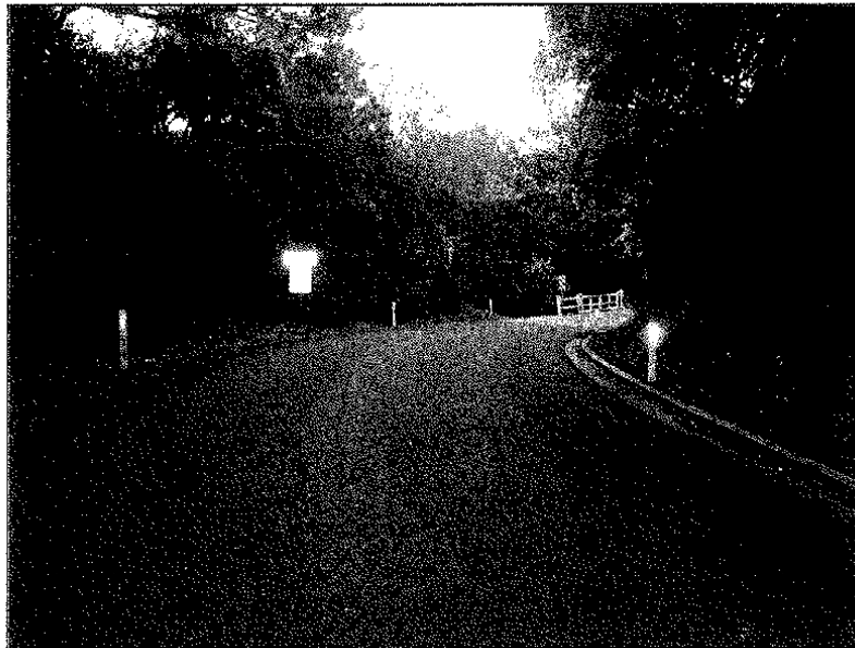
Figure 1 - Eltham Road, south of Gibsons Creek
