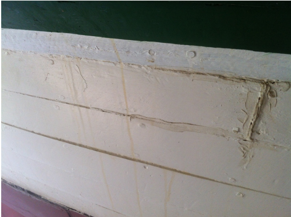
Plate 14: PV Richmond starboard planking. Note repairs to caulking (March 2012).
