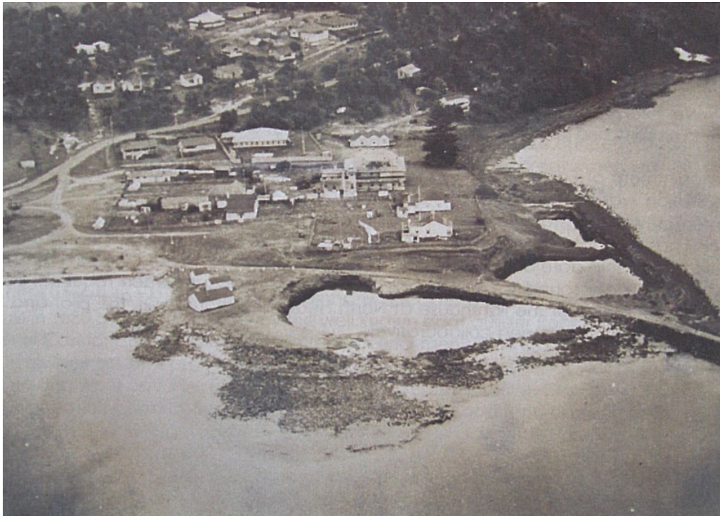
Plate 1: Shaws Bay, showing the Pilot's Cottage and other buildings associated with the Ballina Pilot. Note: 'quarry holes' formed by the removal of columnar basalt to construct the Ballina breakwall. Image courtesy of BSC Records.
