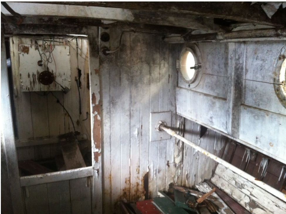
Plate 18: Looking inside starboard cabin/coach-house. Note deteriorated state of paintwork, timber cabin structure and cabin furniture. Exposed frames and hull planking can be seen to the right of the photo. (March 2012).
