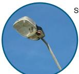
Streetlights across Ballina Shire have been retrofitted with an energy efficient light fitting. These fittings are projected to use approximately 44% less energy to operate, compared to the previous fittings.
