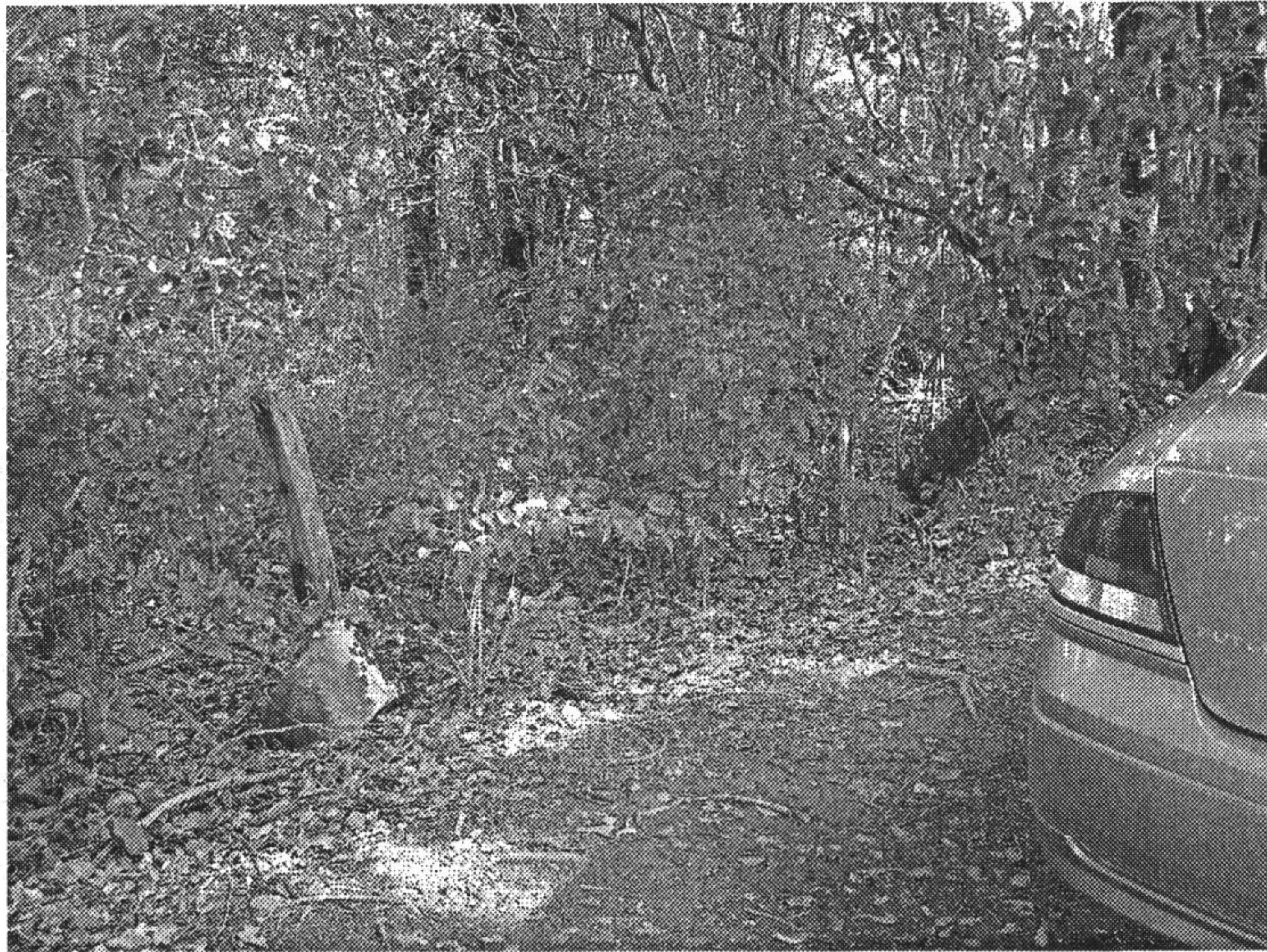
Vegetation and remnants of barbed wire fencing on western (uphill) side of entry point.
