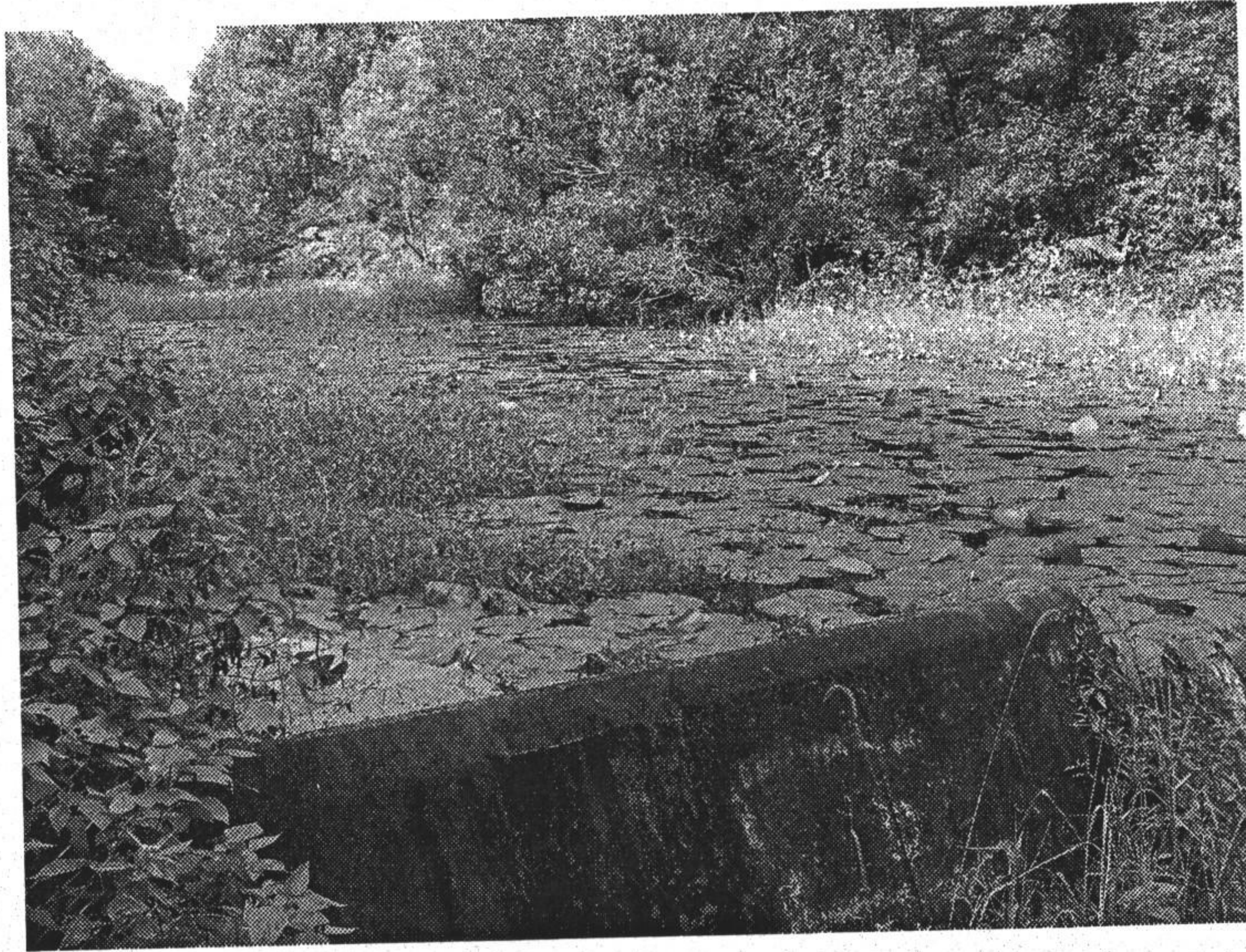
The weir - spillway
