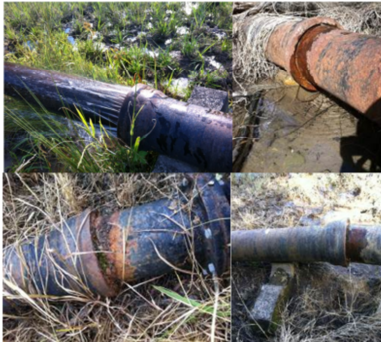
Figure 7.1: Current condition of pipe
