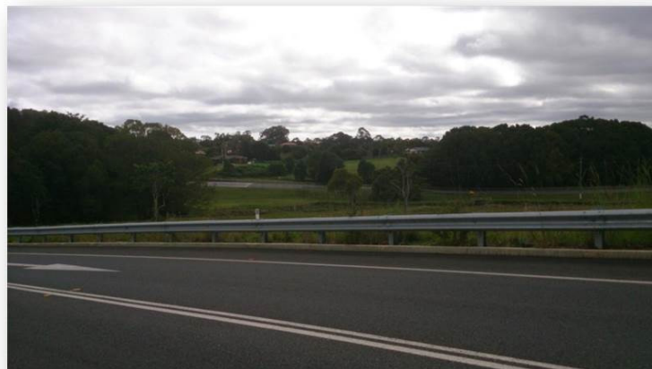
View looking North from the Bruxner Highway exit ramp.
