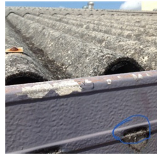
BNM 9 Roof of old building, north east
