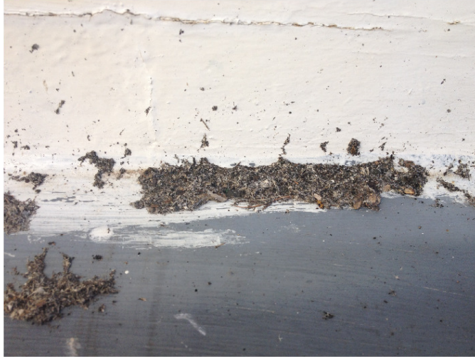
Photograph 3: Asbestos contaminated debris to south elevation top of S.V Richmond (Vessel)
