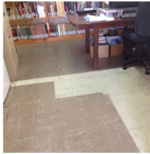
BNM 8 Internal office vinyl floor tiles
