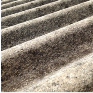
BNM 11 Roof on original section Northern side
