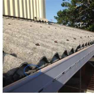
BNM 13 Roof on original section
