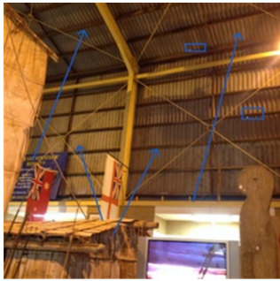
BNM 7 Walls & Roof Internal new section
