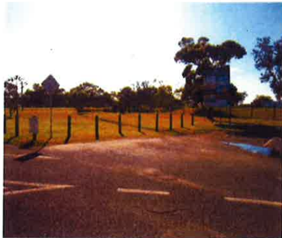
Drainage issues in the existing bitumen carpark
