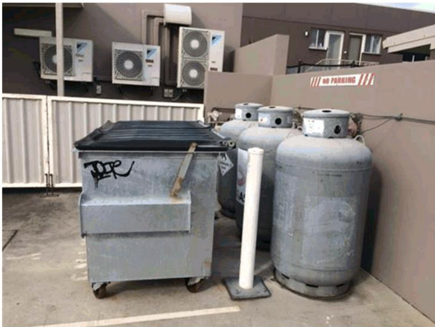
Loading/Unloading area off Park Lane
