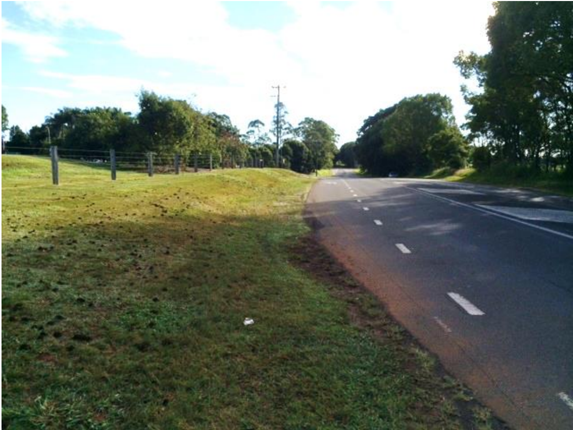
Entry left turn Lane to TAFE and Shoulder where cars park to access sporting events
