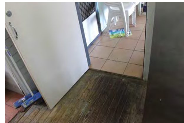
Trip hazards where change of materials occur
