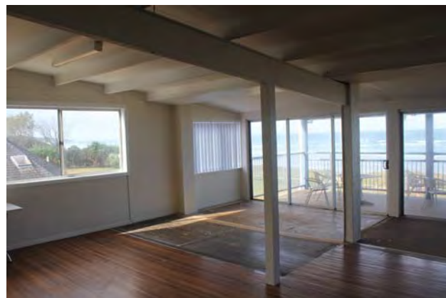
Support columns supporting existing beams
