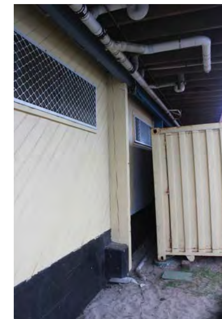
Signs of cracking in support columns / exposed sewer pipes
