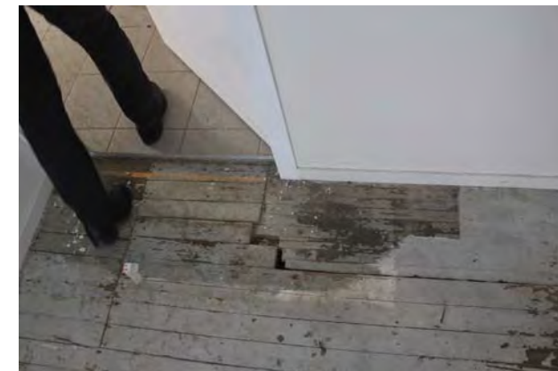
Trip hazards where change of materials occur
