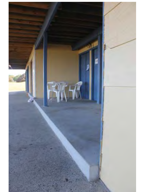
Trip hazard - no equitable access into building
