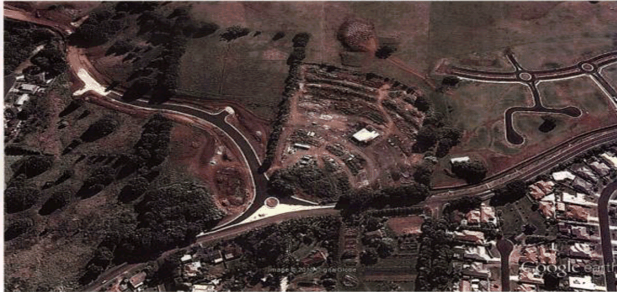
Figure 6. 2011 Historical aerial photograph of site showing disturbance to site due to use as works compound for construction of Plateau Drive.
