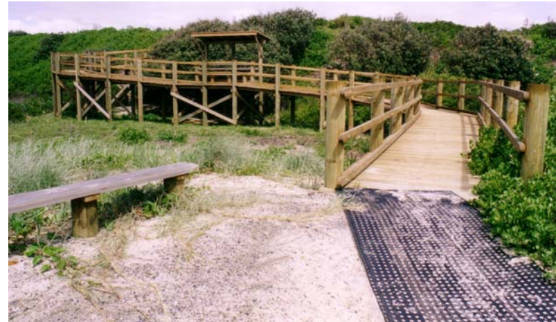
Plate 24: Elevated walkway providing access to the beach. Holey belt can be seen in the foreground.
