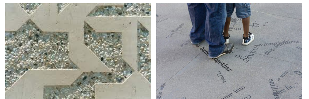
Images of sandblasted concrete and pavement art
