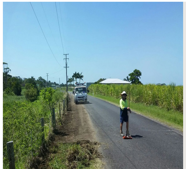
Example of a rural road with a spray seal surface.
