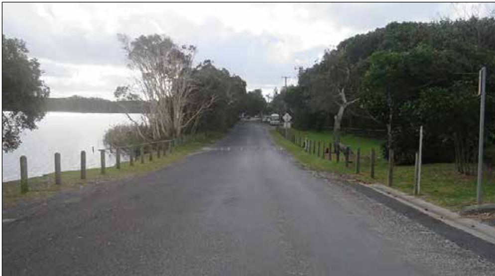
Figure 18 – The eastern foreshore of Lake Ainsworth has disappeared with water at some places lapping at the roadway. Camera direction is north from the surf club.
