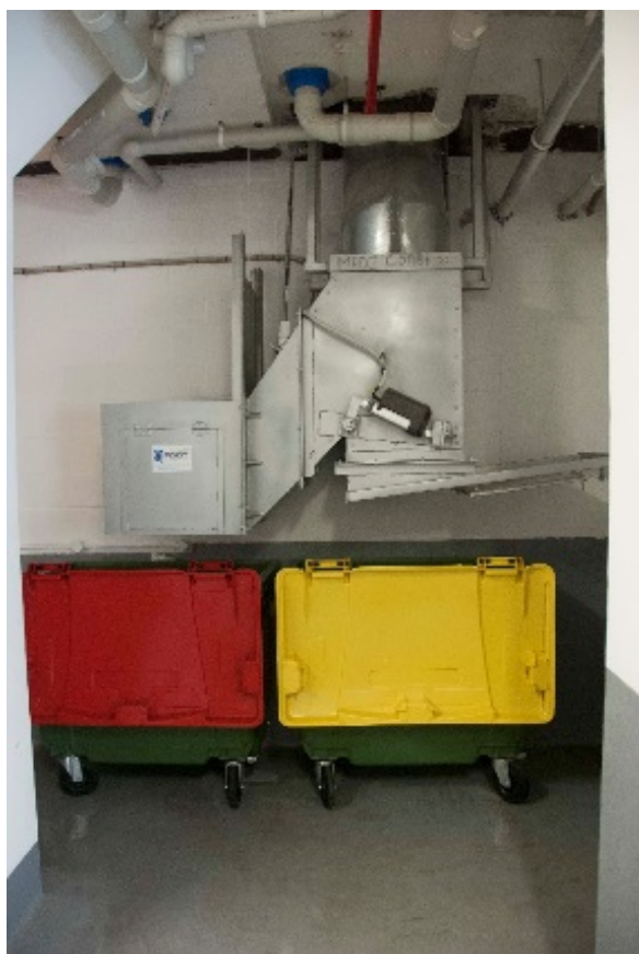
Example of a diverter chute system (waste and recycling) using 660 L bins (Photo: Andrew Quinn)
