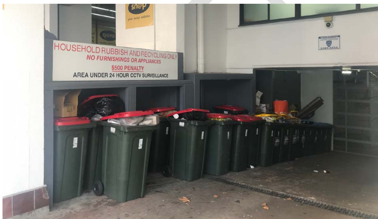
Mixed use residential waste collection point Bondi Junction (Photo: Elton Consulting)
