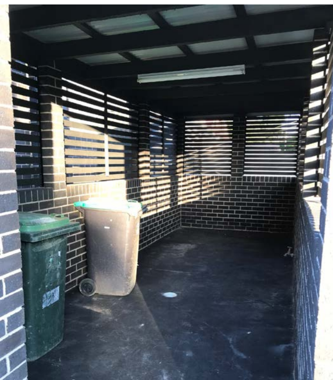
Bin storage with screening, robust construction and washing facilities (Photo: Penrith City Council)
