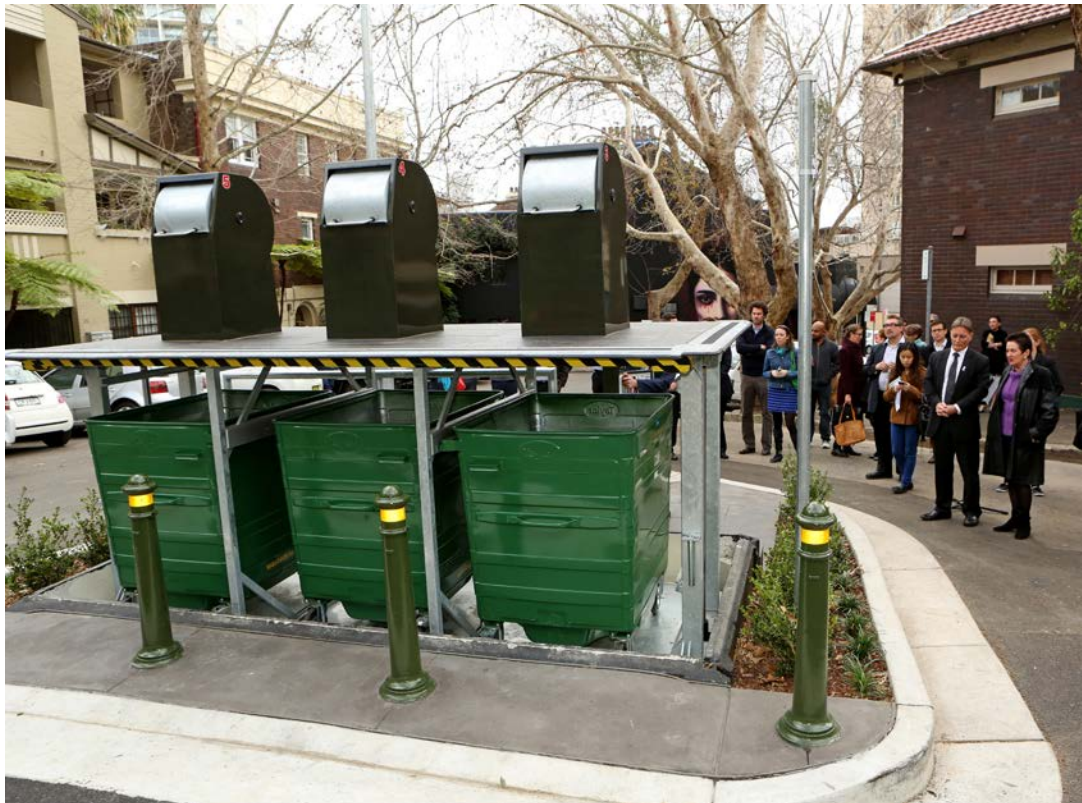
Example of an underground bin system in Sydney used by the residents living in residential flat buildings in the surrounding area (Photo: Andrew Quinn) Approval to use this photo?
