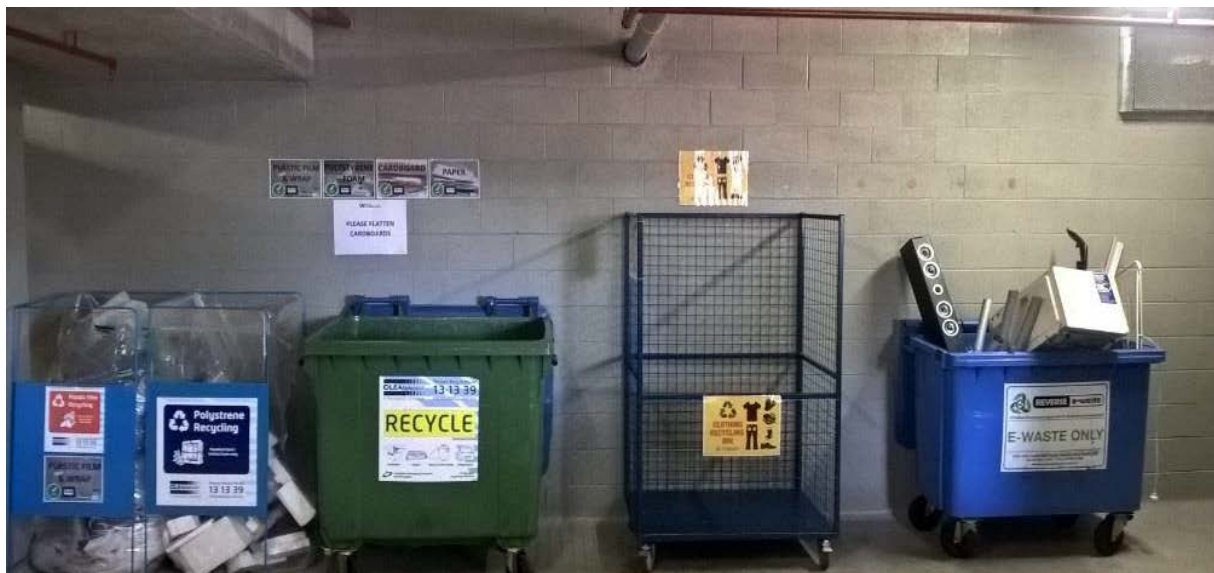
Problem waste storage area for e-waste, polystyrene, clothing and recyclables in the basement of a high-rise building – (Photo: City of Canterbury Bankstown)
