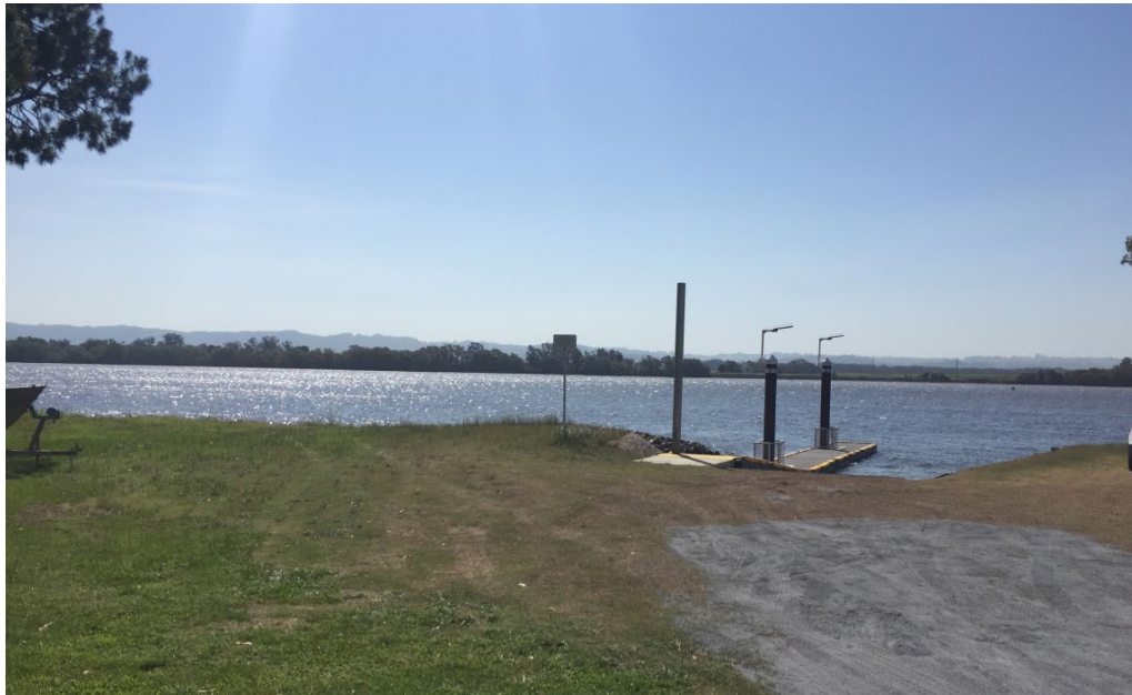
Fig Two: New boat ramp with floating dock. Keith Hall Lane.
