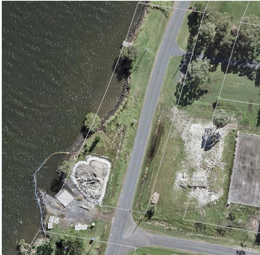
Fig One: The subject site overlaid by the community land parcel Lot 1 DP958042 and Keith Hall Lane, formed road.
