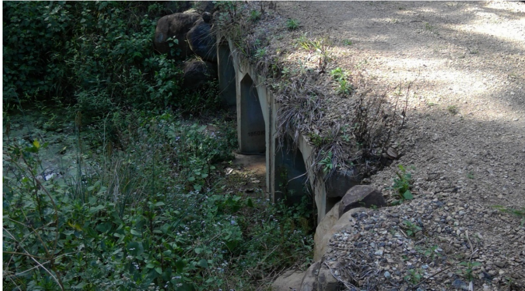
Figure 10: Concrete Culvert Water Crossing
