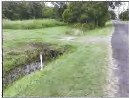
Photo 5 - Table drain within the road reserve.
