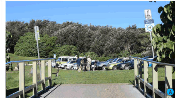
Above: Existing boardwalk component of the shared pathway that connects the Pat Morton Lookout Precinct to Lemnox Head Village Centre.
