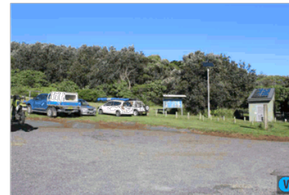
Above: General view of the carpark and built elements with a vegetated backdrop
