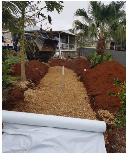
Figure 2 – Installation of OSSM
