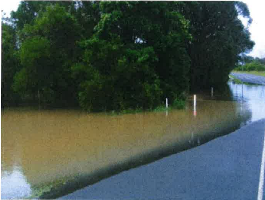
View looking north along Newrybar Swamp Road at existing pipe crossing. Note water build up on western side to our property and driveway access point due to lack of appropriate drainage infrastructure under Newrybar Swamp Road.
