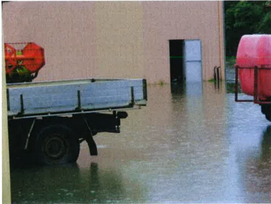
View towards shed outbuilding from the house verandah.
