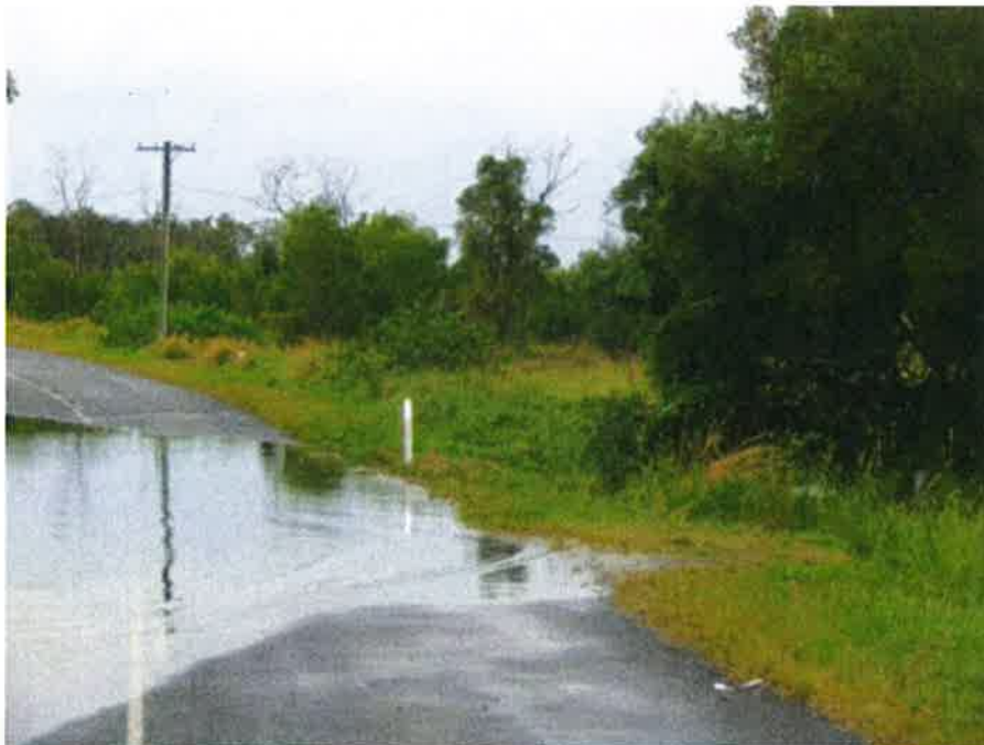
Note minimal water on eastern side of Newrybar Swamp Road compared to western side.
