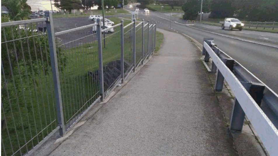
Photo 28 – Hill Street, shared path, barrier fencing, guard rail with timber board
