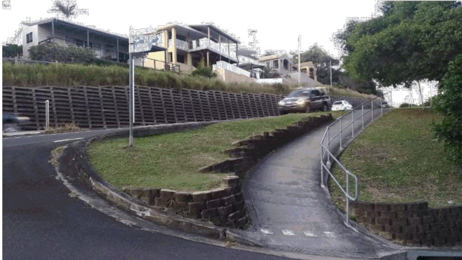
Photo 27(b) – Compton Drive at Hill Street intersection, footpath
