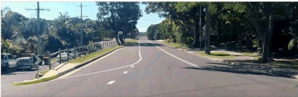
Photo 14 – CH 950 – View to the EAST – Intersection with western end of Cronulla Street
