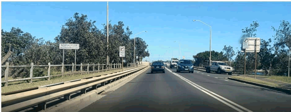
Photo 40 – CH 75 – View to the WEST – Intersection with The Serpentine
