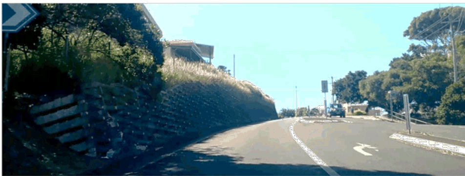
Photo 6 – CH 350 – View to the EAST – Intersection with Compton Drive
