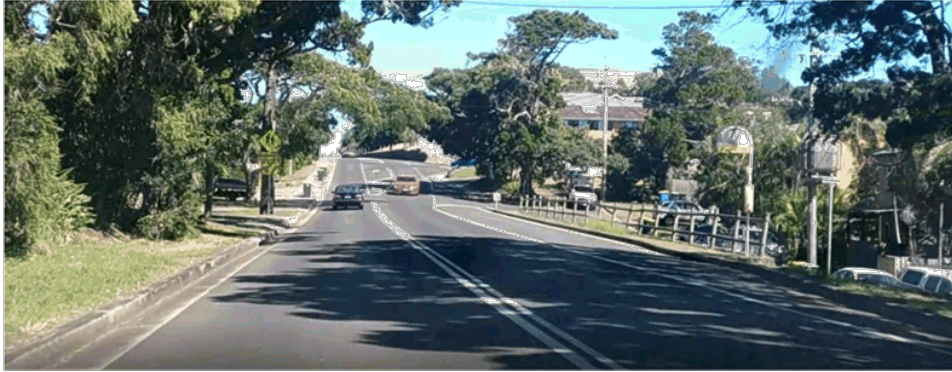
Photo 27 – CH 1,000 – View to the WEST – Bus stop
