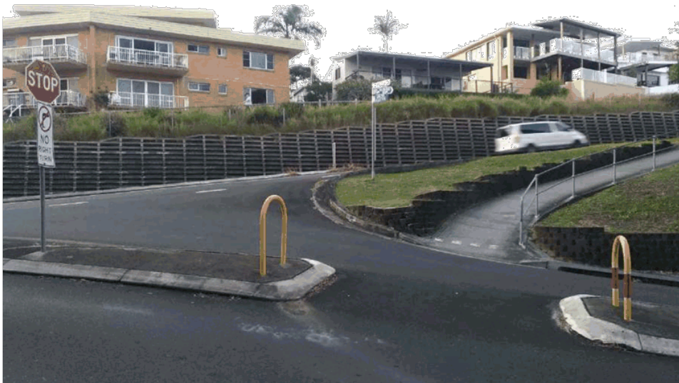
Photo 27(a) – Compton Drive at Hill Street intersection, refuge island
