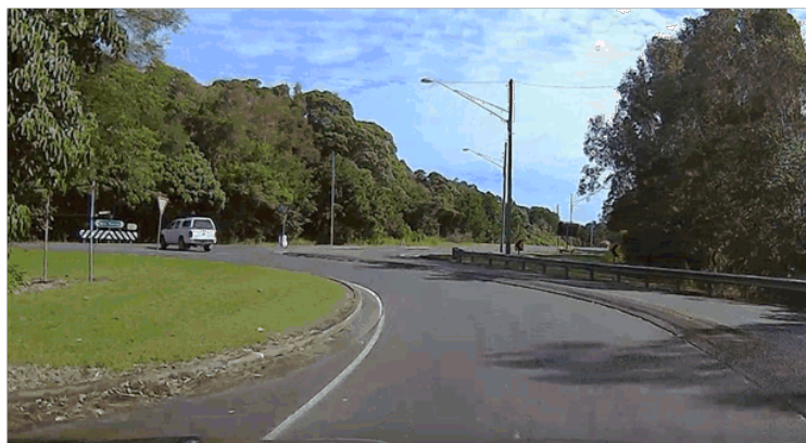
Photo No. 3: Existing westbound approach to intersection – single lane. Note narrow lane eastbound side
