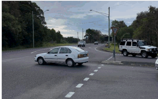
Photo No. 5: Location of hold line, set well back from through lane
