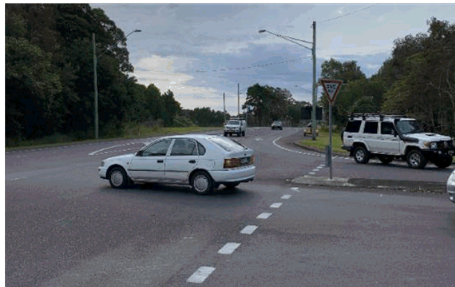
Photo No. 2: Location of existing hold line, set well back from through lane
