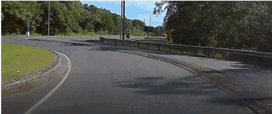
Photo No. 4: Lack of visibility of median – Byron Street
