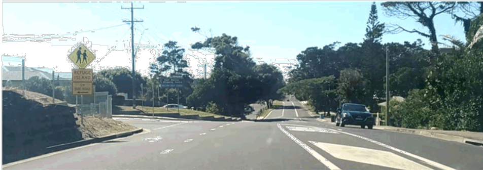
Photo 12 – CH 900 – View to the EAST – Intersection with Manly Street
