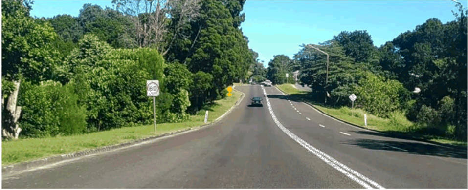
Photo 24 – CH 1,300 – View to the WEST – Reinforcing 60 km/h speed zone sign
