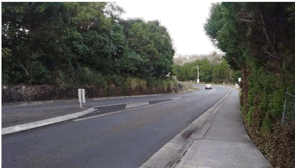
Photo 27(c) – Compton Drive, footpath
