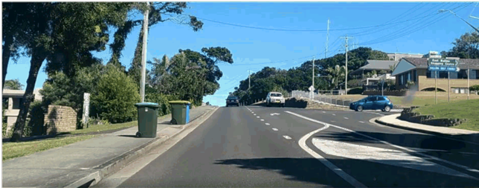
Photo 29 – CH 925 – View to the WEST – Intersection with Manly Street
