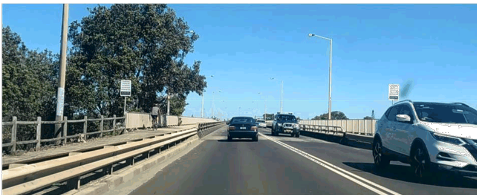
Photo 41 – CH 0 – View to the WEST – East end of Missingham Bridge
