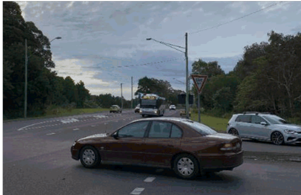
Photo No. 1: Sight distance to the north with turning vehicle (note through vehicle beside rear of bus, still obstructed with stopped vehicle in front of hold line)
