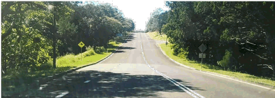
Photo 17 – CH 1,200 – View to the EAST – AUR for the intersection with Suvla Street
