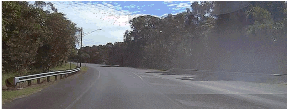
Photo No. 1: Condition of line marking
