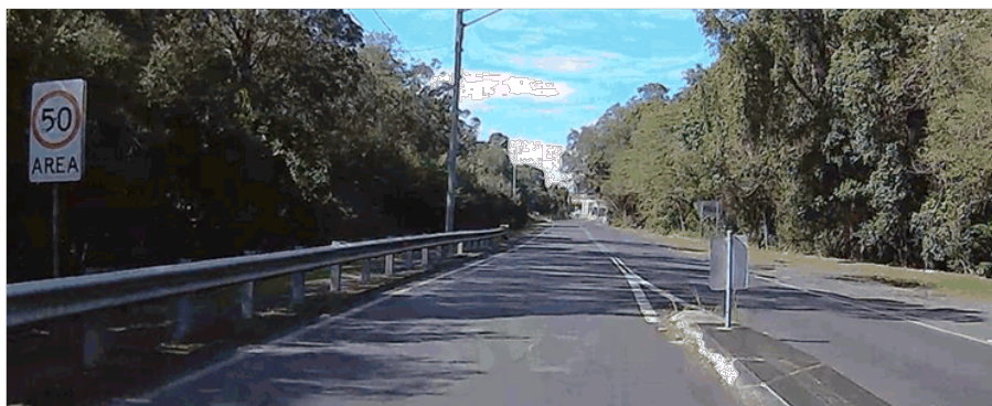
Photo No. 3: Condition of pavement marking at 50 zone
