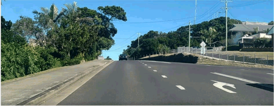
Photo 30 – CH 900 – View to the WEST – Intersection with Manly Street
