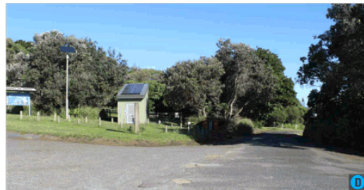
Above: Exit from the car parking area between existing native vegetation. Weathered pavement surface and eroded swale drain.
