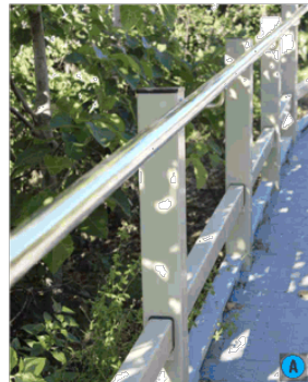
Above: Existing boardwalk construction
