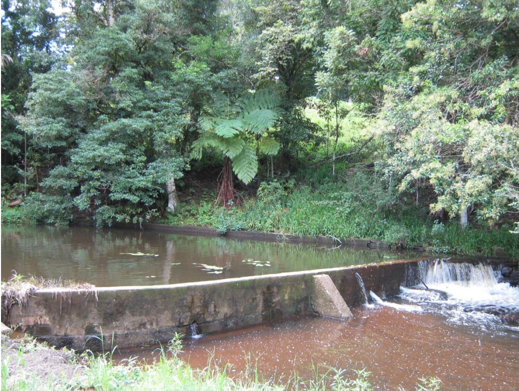
Plate 9: Looking across the weir from zone 2 to zone 4.
