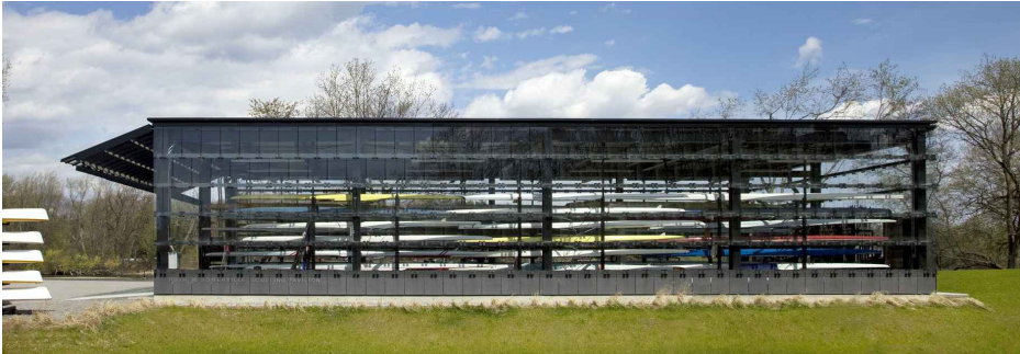
Above: Watercraft Storage - Example of a low-set/accessible watercraft storage area (Source: Inhabitat - Boathouse by Anmahian Winton Architects). A simple structure with roof, internal shelving and a combination of mesh and solid sides. Wide access doors provide easy boat maneuverability. This example shows the potential of a higher cost option.
