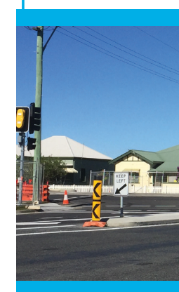
River Street Duplication (Stage 2 – Henry Philp Avenue to Tweed Street)
