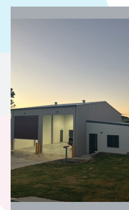
Completed Lennox Head Rural Fire Shed
