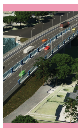
Commenced preliminary River Street Duplication (Duplicating Fishery Creek and Canal Bridges)
