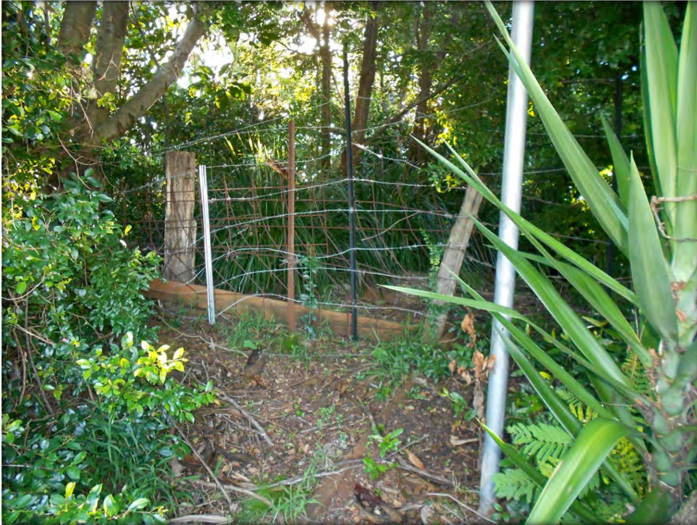
Figure 14: Vandalised fencing at Kim Court to be replaced
