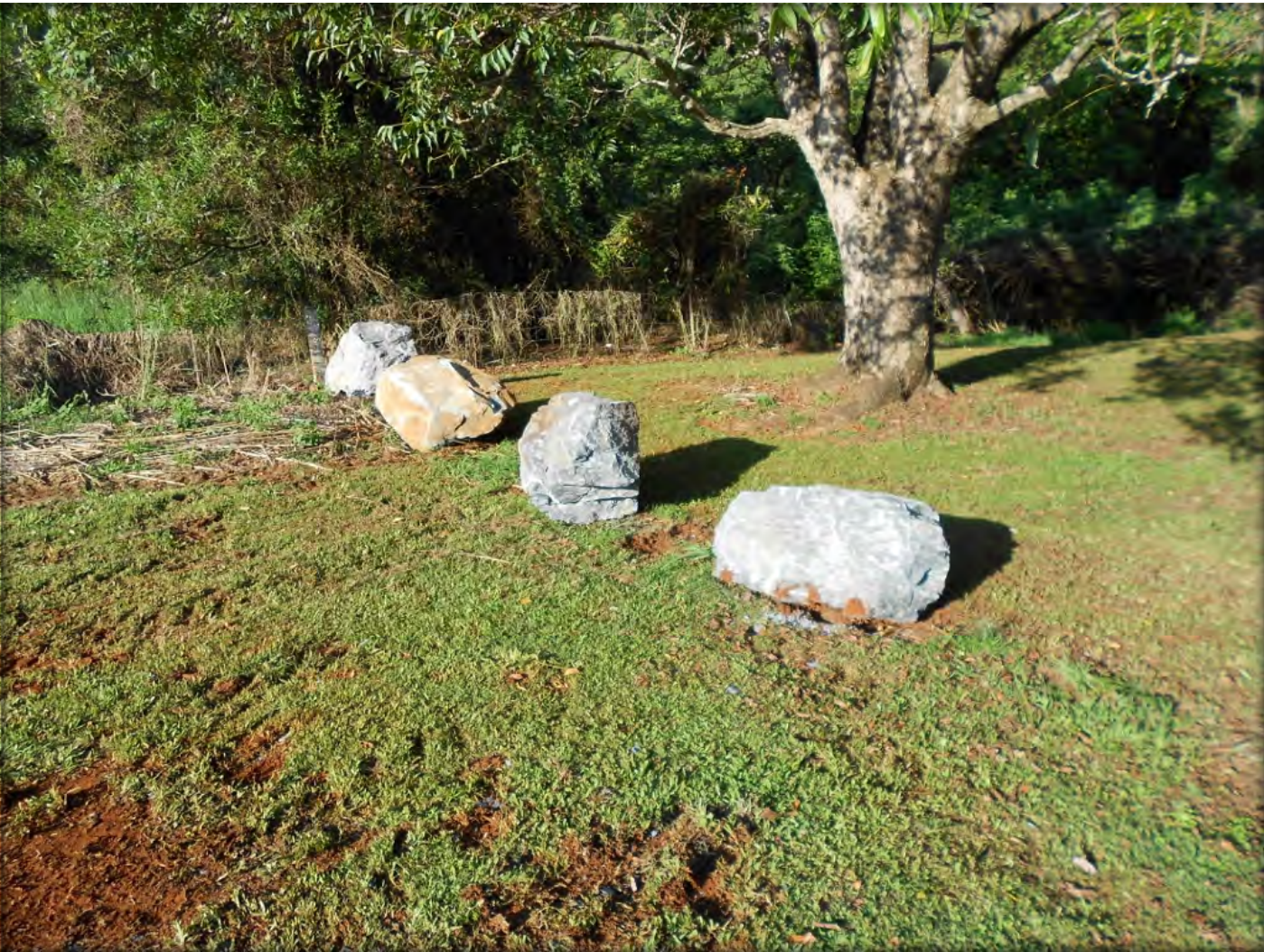
Figure 17: Rock bollards to prohibit vehicles at Johnstons Road
