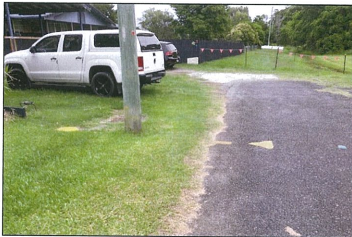
Photo 12 - Existing street hydrants located in Fitzroy Street.
