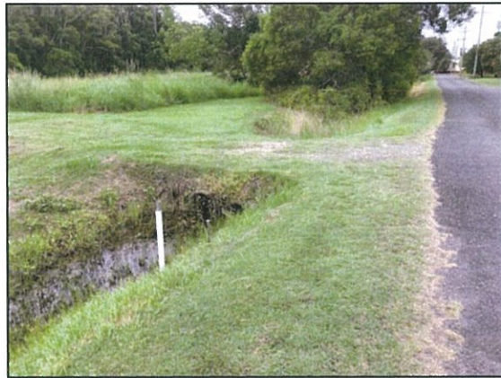
Photo 5 - Table drain within the road reserve.
