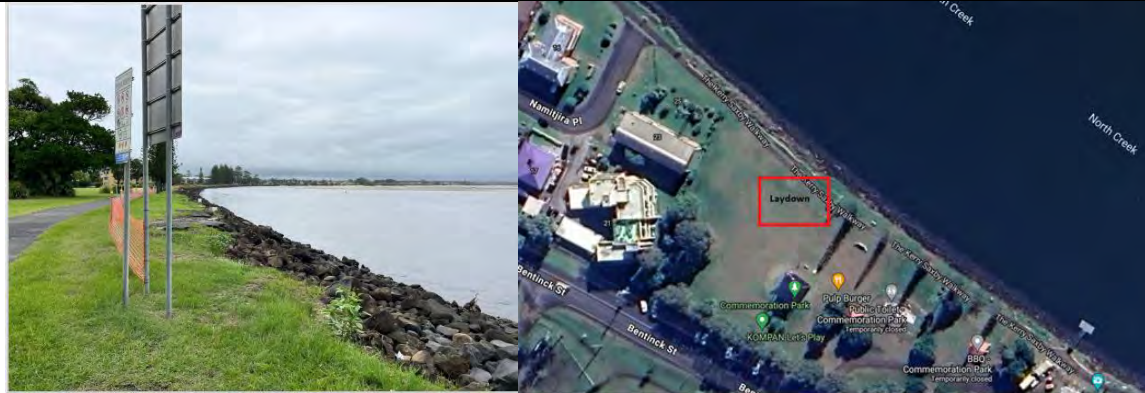
Site 2.5: View looking northwest at Site 2.5 located on USL and within Commemoration Park (left). Laydown area within Commemoration Park (right).
