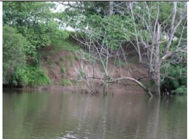
Slumping causing tree fell into the River, Wilsons River.
