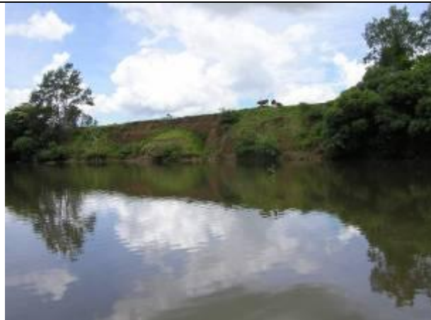
Severe bank slumping, Wilsons River.
