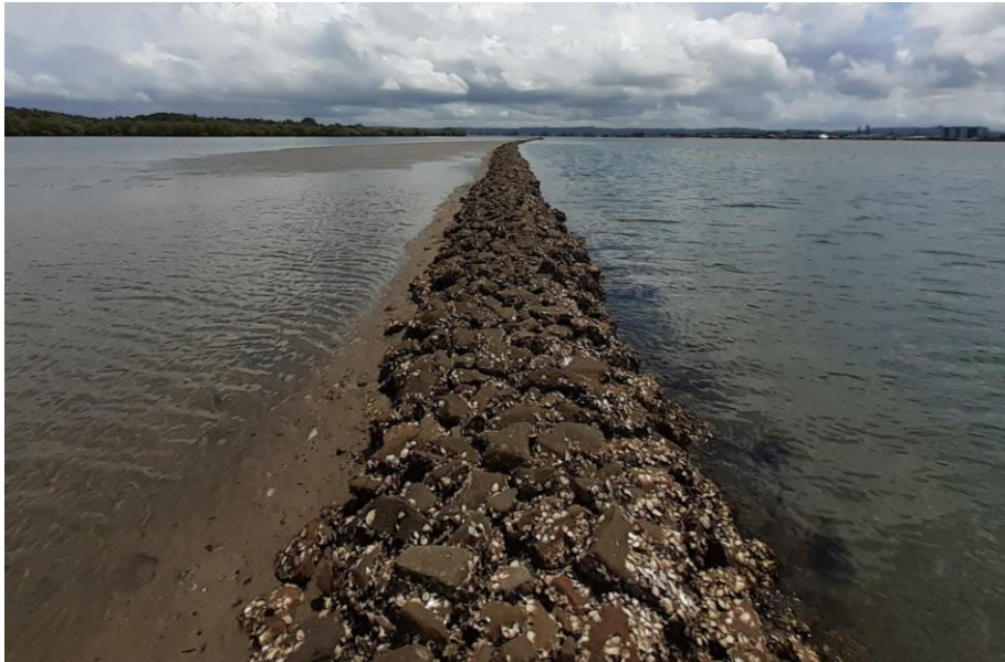
Figure A.25: Mobbs Bay training wall looking west
