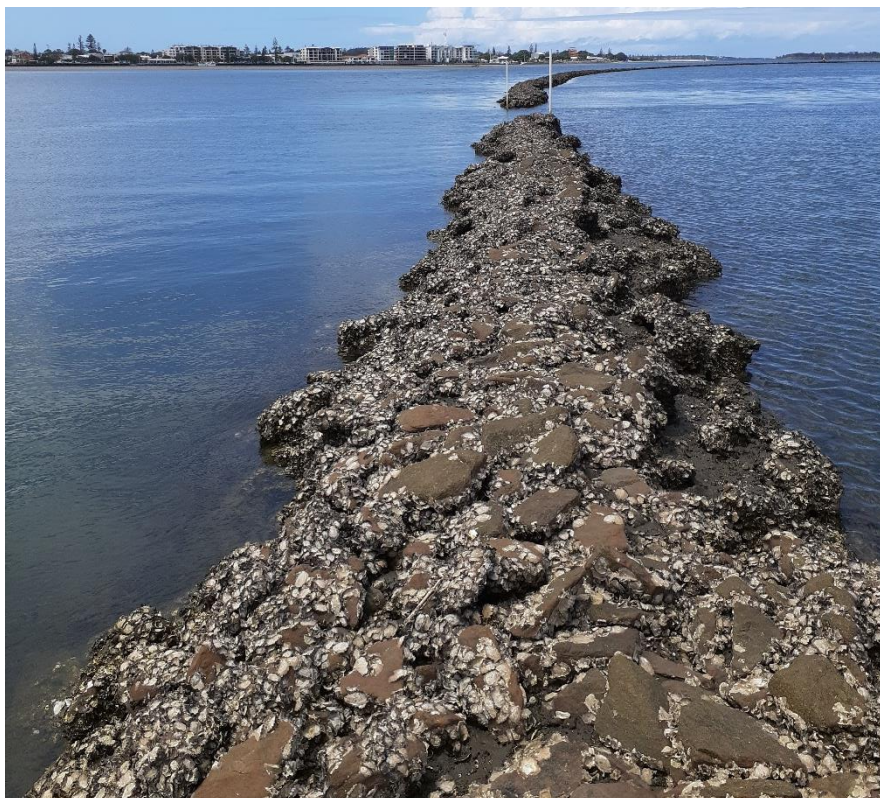
Figure 4.8: Mobbs Bay training wall looking east
