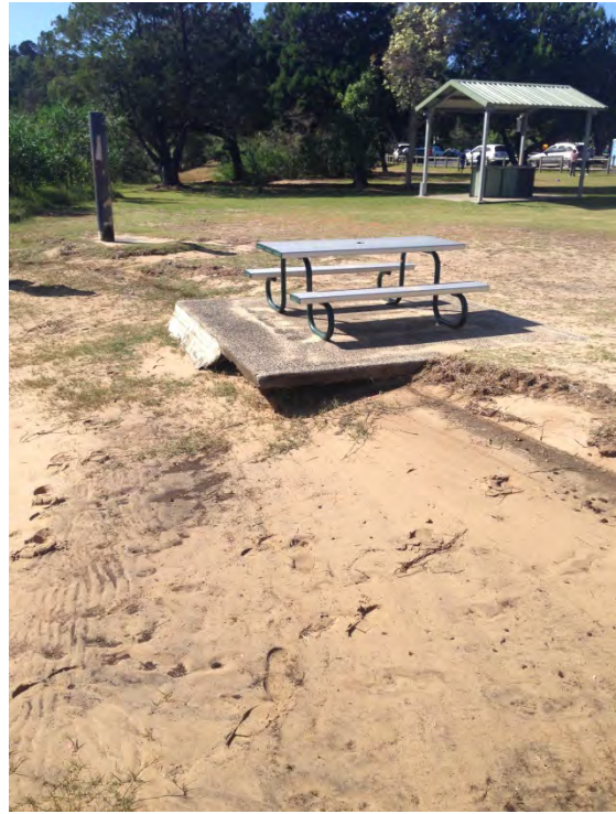
Photo 4: Erosion to be remediated by beach nourishment at South Pop Denison Park Beach
