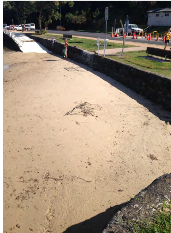
Photo 12: Western Foreshore Ramp
