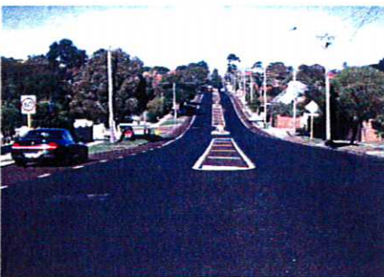
PAINTED MEDIAN TREATMENT
