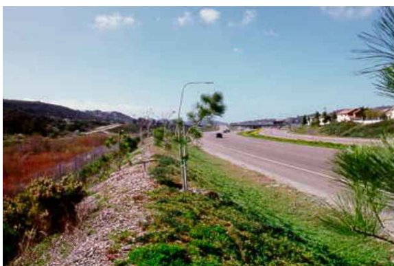
Example of earth mound barrier
