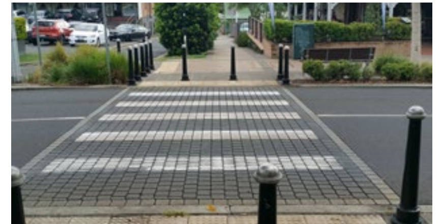
Main Street beautification works completed in 2010-2011
