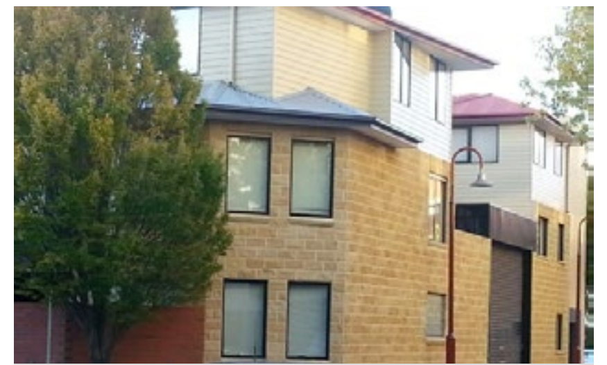
example of three storey residential development
