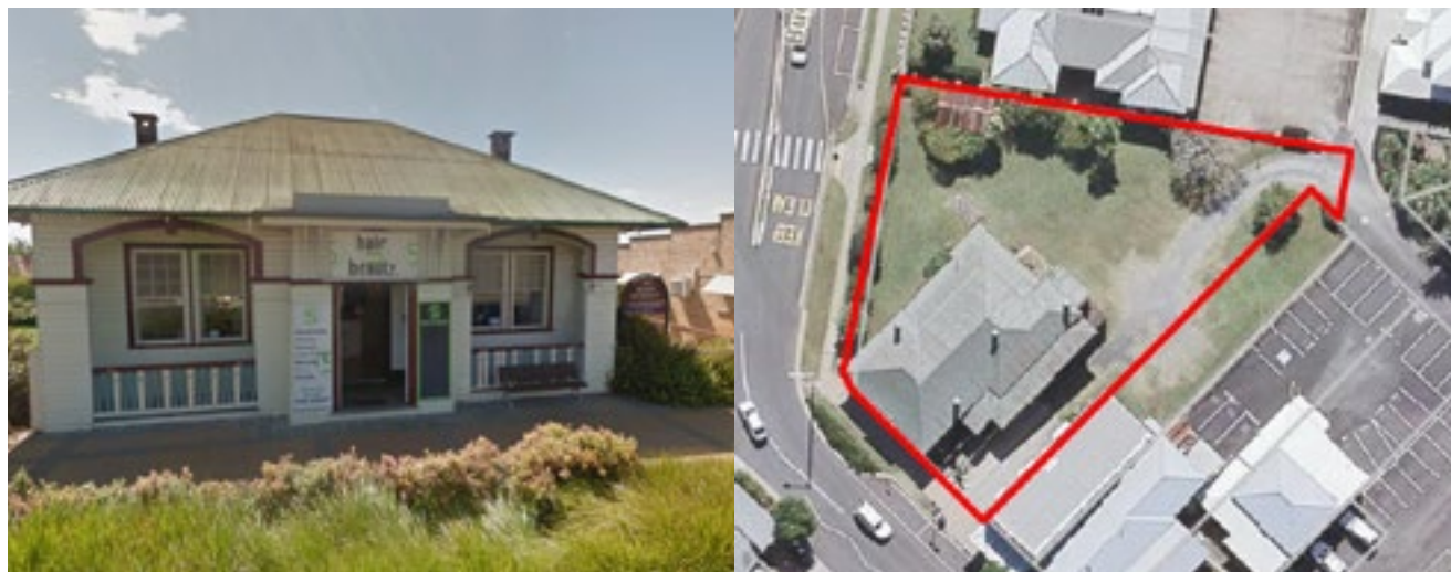
70 - 74 MAIN STREET, ALSTONVILLE
