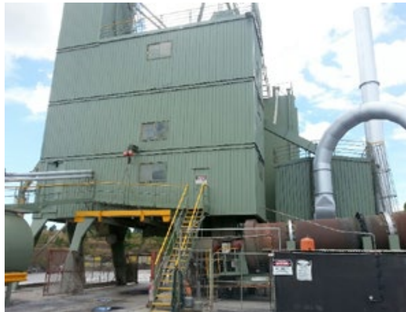
Asphalt plant within Tuckombil Quarry Site
