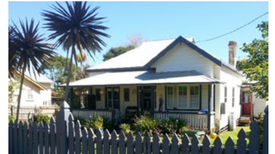
33 Main Street, Alstonville
