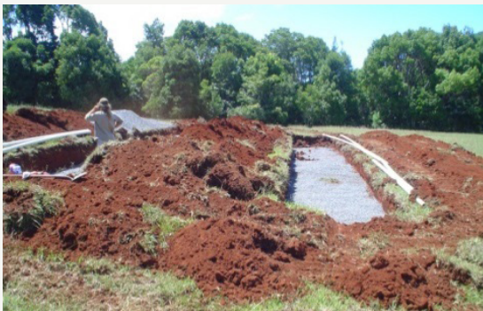
Figure 13: ETA bed under construction.
