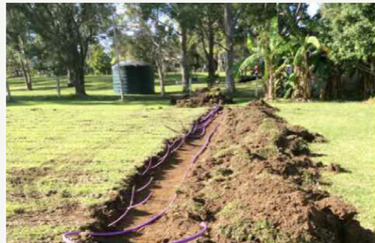
Figure 18: Sub-surface irrigation system under construction.
