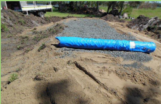
Figure 15: Sand mound under construction.
