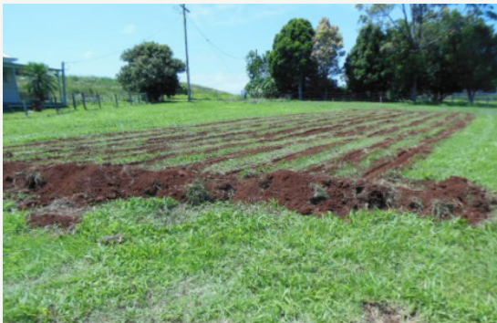
Figure 17: Sub-surface irrigation system under construction.
