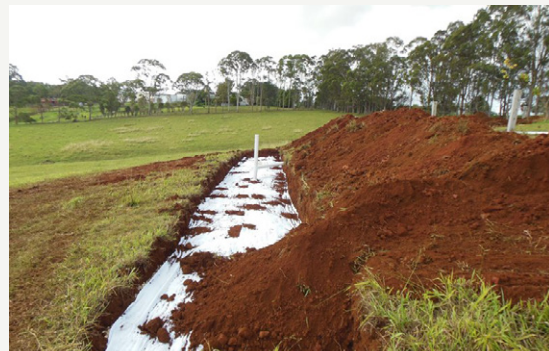
Figure 14: ETA bed under construction.
