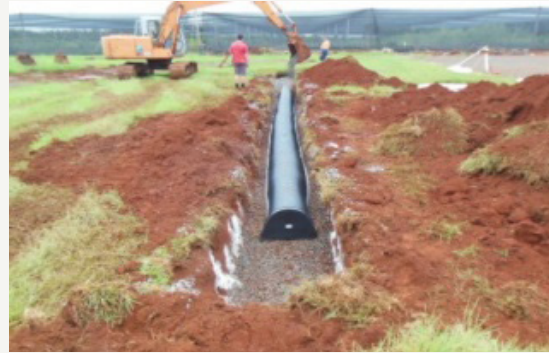
Figure 12: Absorption trench under construction.
