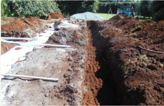
Figure 11: Absorption trench under construction.
