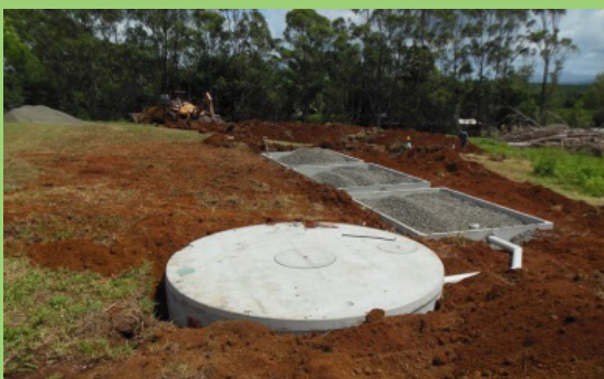
Figure 10: Reed bed under construction.
