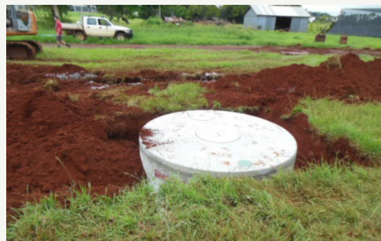
Figure 2: Septic tank installation
