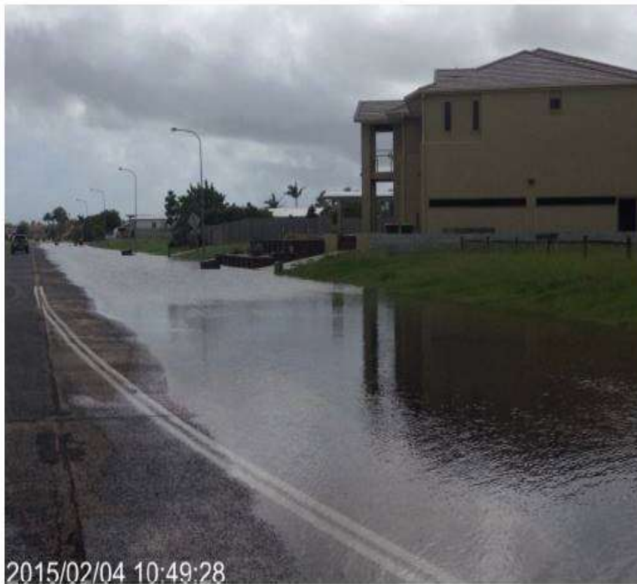
Plate 4: Tidal inundation southern end of Burns Point Ferry Road
